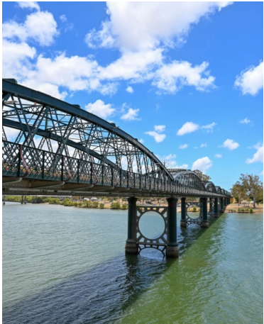
Bundaberg Bridge 6 Jenny Shackles
